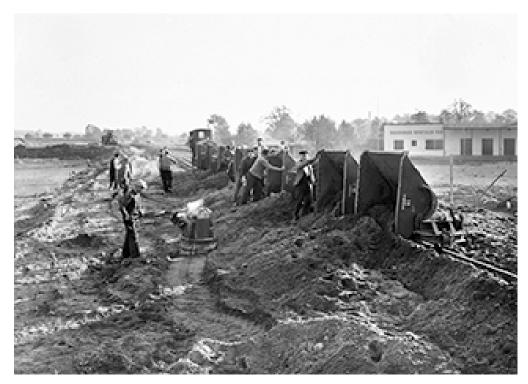
Fig. 2: *Reichsautobahn* under construction, in Radeburg (Saxony), 1937; a four-metre-high dam is built with manual labour (SLUB/Deutsche Fotothek, Walter Möbius)
