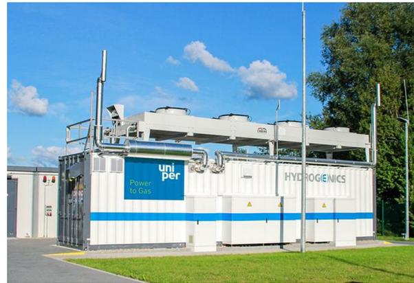
**Fig. 4.** Typical containerized PEMWE system in the 1 MW power range at Windgas Hamburg, Reitbrook project site. (Copyright ©Uniper SE).
